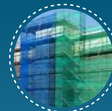
Buildtech (Construction Textile)
