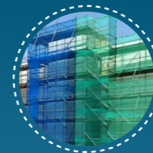
Buildtech (Construction Textile)
